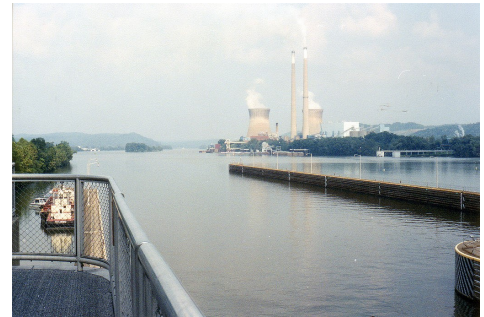
Pleasants Power Station | FirstEnergy
